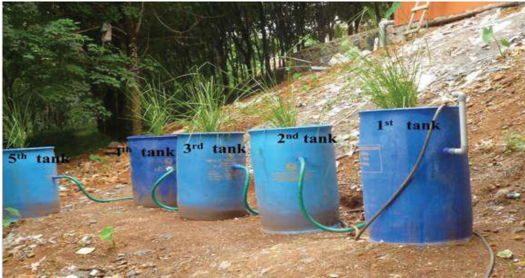
(a) Immediately after construction
